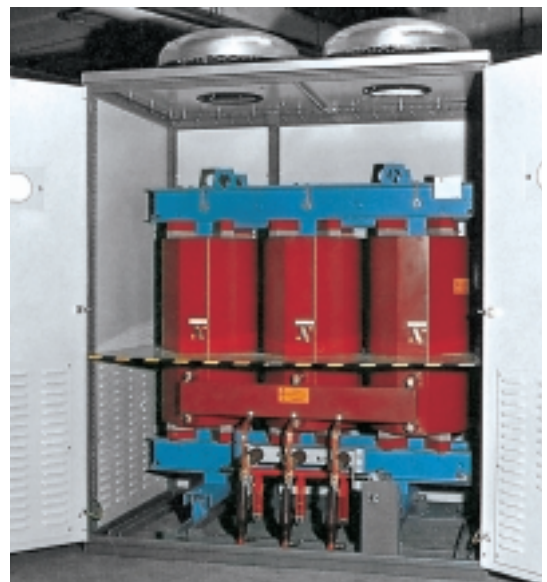
Fig. 54: GEAFOLE transformer in protective housing to IP 20/40
