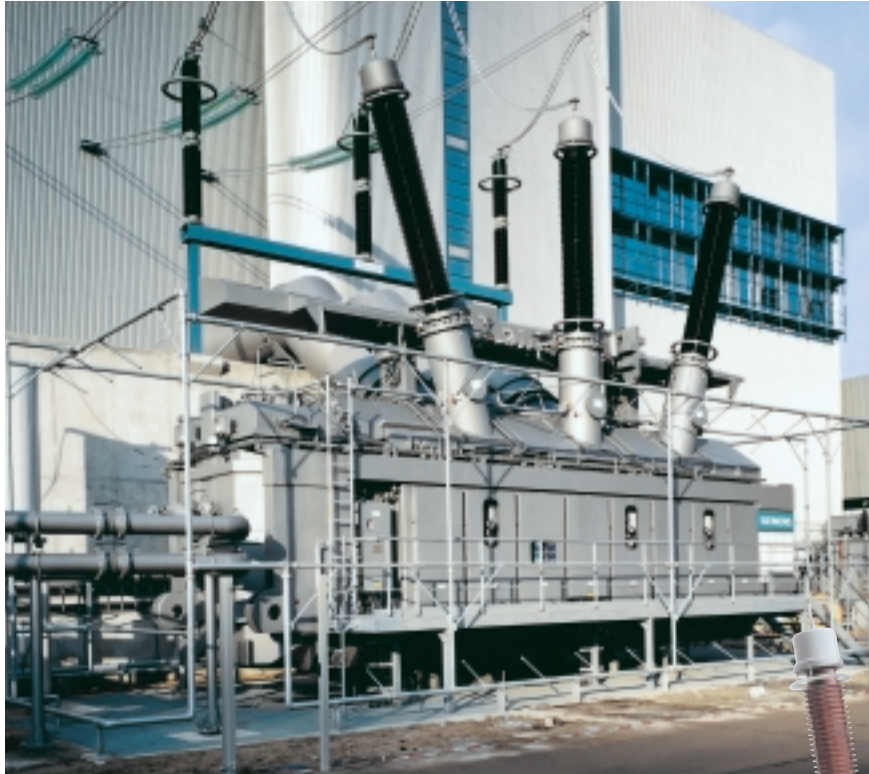
Fig. 43: Coal-fired power station in Germany with two 850-MVA generator transformers: Low-noise design, extended setting range and continuous overload capacity up to 1100 MVA
